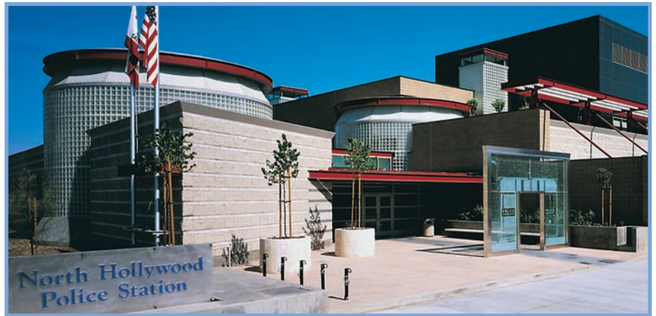
North Hollywood Police Station, N. Hollywood, CA Architect: Meyer & Allen Associates // ARGUS® Pattern and HEDRON® Corner Block
